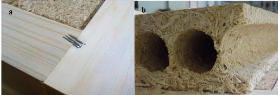
**Fig. 1.** Frame joint between fir wood elements (a) and hollow extruded chipboard (b)
